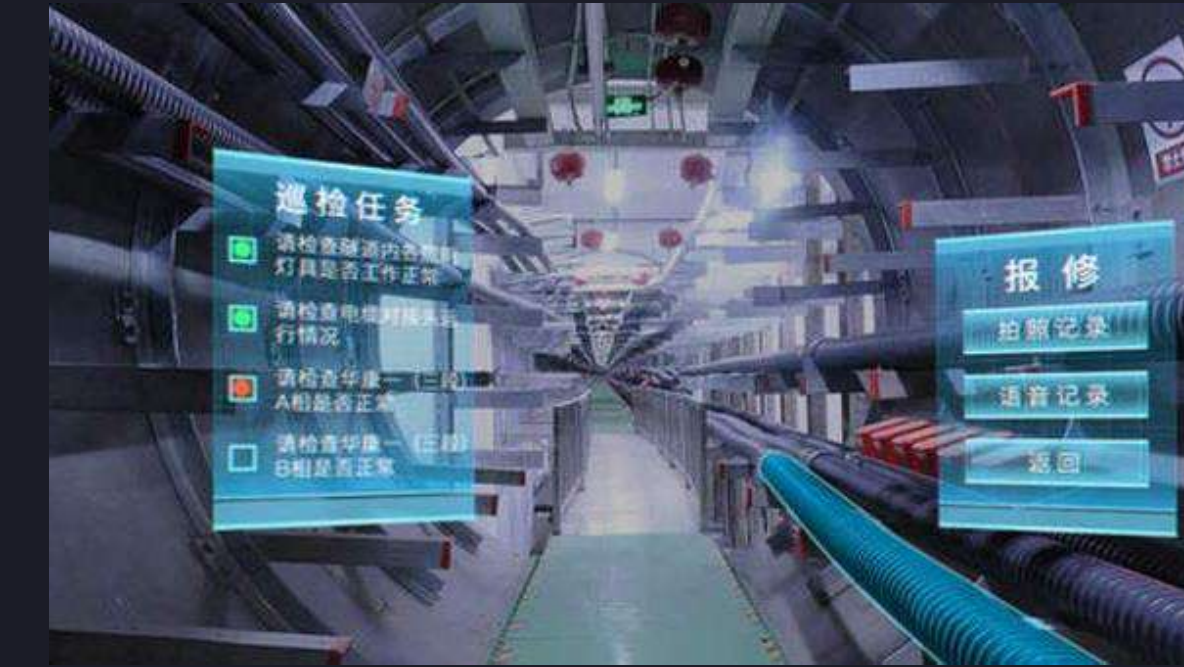
On-site intelligent inspection
